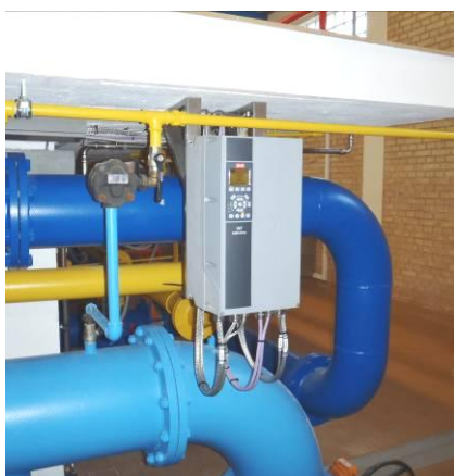
Frekvensomformer for rentvands- pumpe 4
